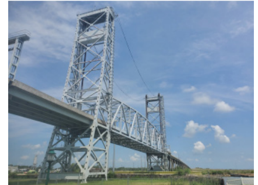
Figure 1. Ellender Ferry Bridge, SR 27, Calcasieu Parish, Louisiana
